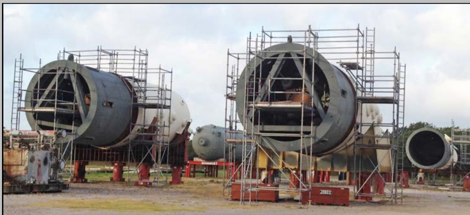
DISMANTLED AND READY TO MOVE
