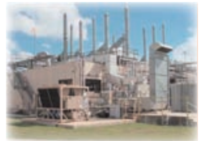
High Pressure Lab Building 10 Cells Totaling 3,700 SQ. FT.
